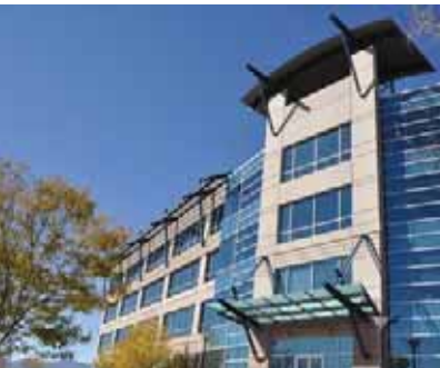
Church Ranch is already a well-established district with highly visible landmark developments like the Westin in the Westminster Promenade and Circle Point offices.
